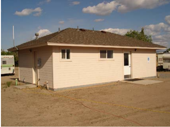
The west bathhouse features two restrooms, two showers, and a laundry room.
